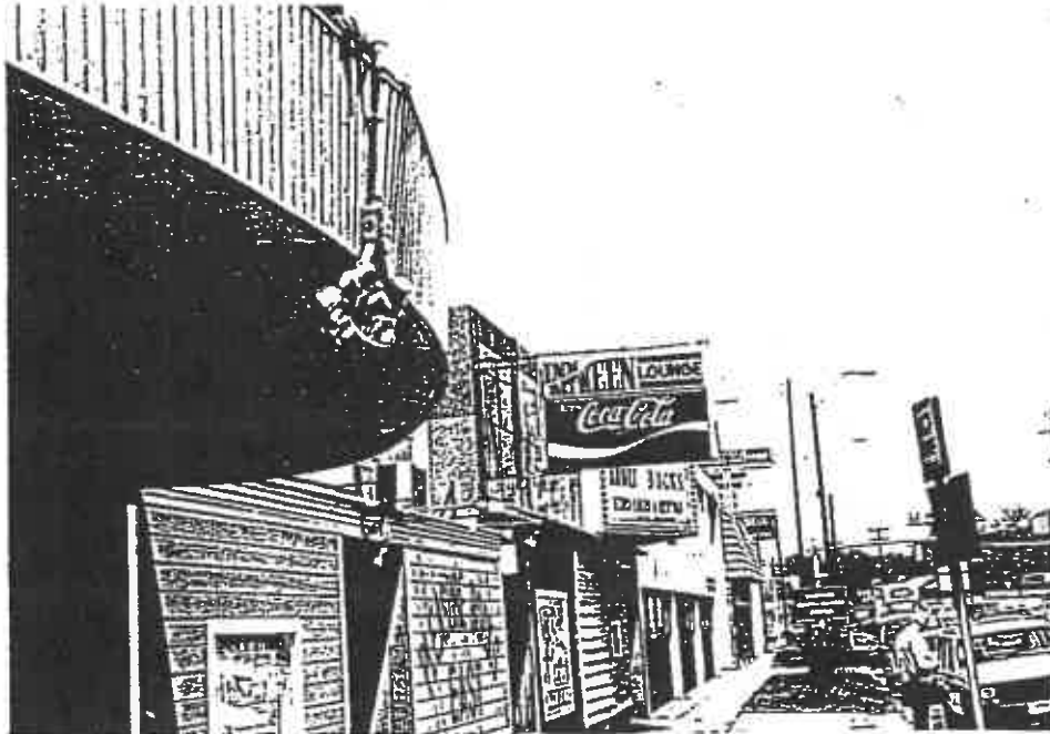
Out of proportion signs or signs that materially obscure the surface of the building shall not be permitted
