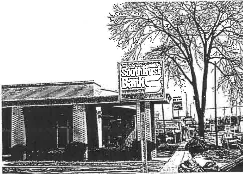
Example Of A Free Standing Sign Which Meets The Guideline Requirements.
