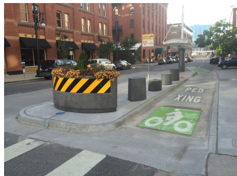
Floating bus islands allows for safer and more efficient boarding and alighting (Denver, CO)
