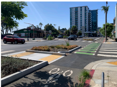
Unsignalized intersection featuring protective buffers for pedestrians and bicyclists (San Diego, CA)
